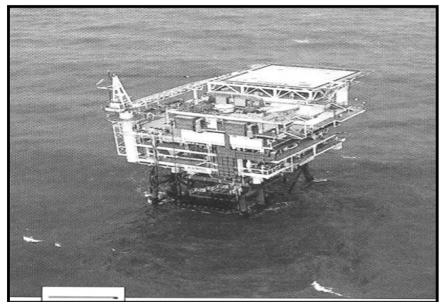
Kumul Oil Terminal, Gulf Province, Oil is piped to this terminal where it is taken away by ships.
