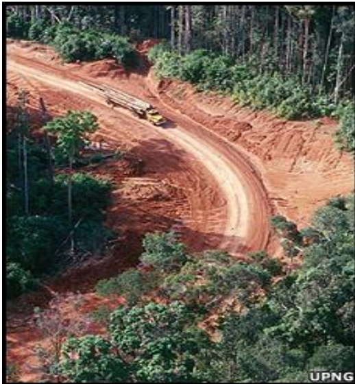
A newly cut road for transporting timber
