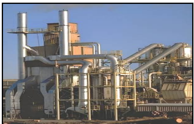
Clean Air Scrubbers can help Reduce the Air Pollution Caused By Burning of Coal
